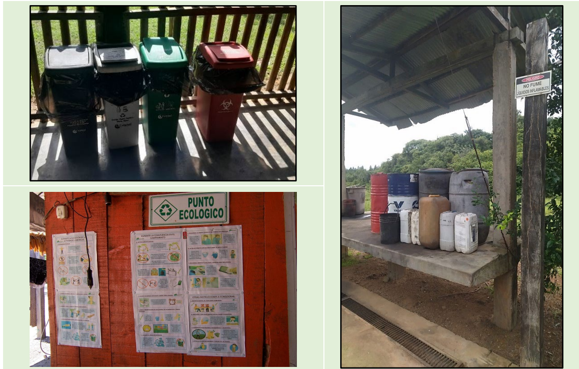
Image 11. Signs used in the projects for proper waste management and disposal. The oil and fuel handling areas are isolated and have channels for collection in case of any type of spill.
